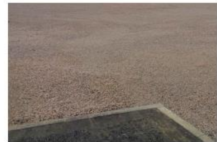
HEAVY DUTY ROAD CONSTRUCTION (SURFACE COURSE), HARDCORE SURFACING & KERBING
