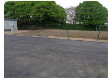
HEAVY DUTY ROAD CONSTRUCTION (BINDER COURSE)
